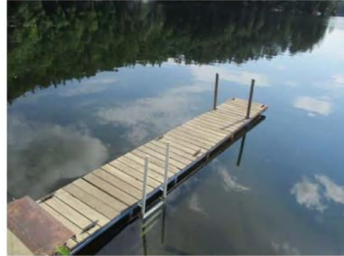
Image of dock that is normally 18 inches above the water
